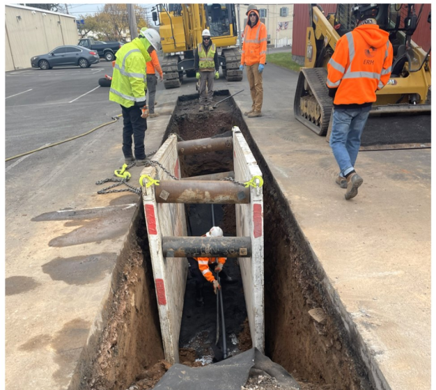
Construction crew trenching on Meyers Way to lay the conveyance piping for the treatment system.
